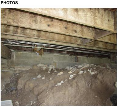
12. The mechanical flexible heating duct under the main floor has the outer cover and inner insulation ripped open. If the ducting is being used, we recommend that they should be replaced where the ducting has been compromised.
